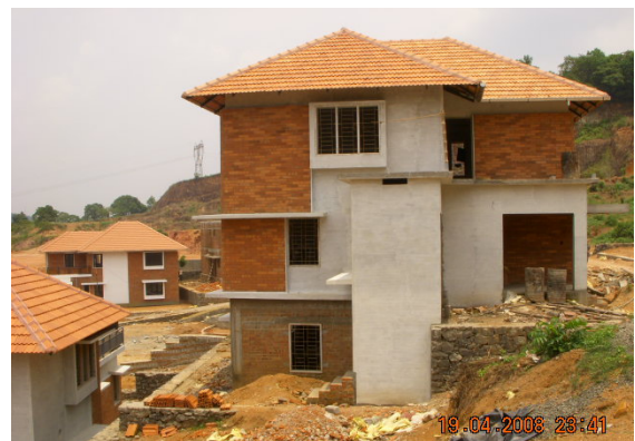
Side view- with cellar floor and first floor
