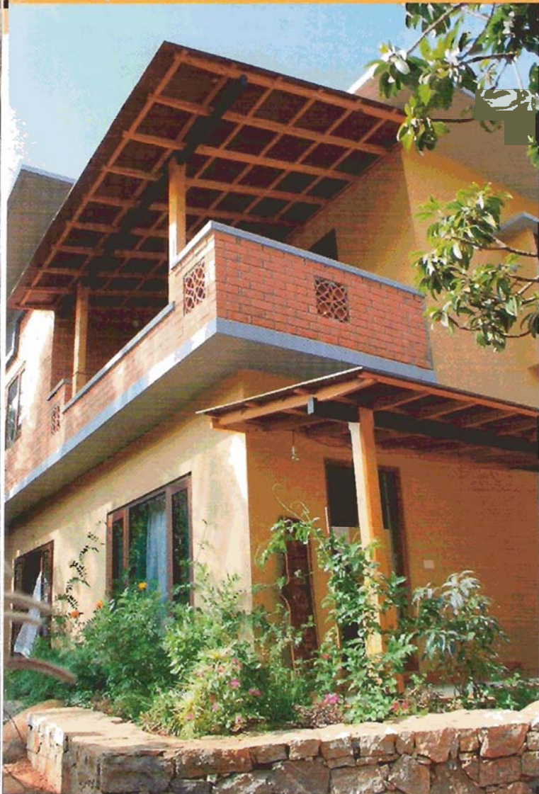
Exposed brick and stone is used in the exteriors while stone, clay and wood are used to dress up the interior spaces
